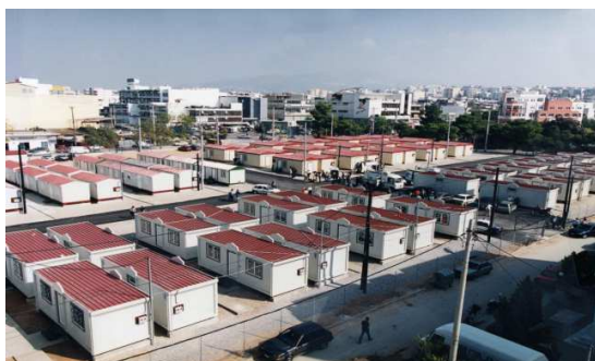
Fig. 6. Modular prefabricated houses for affected regions, (Nikos, 2016)
